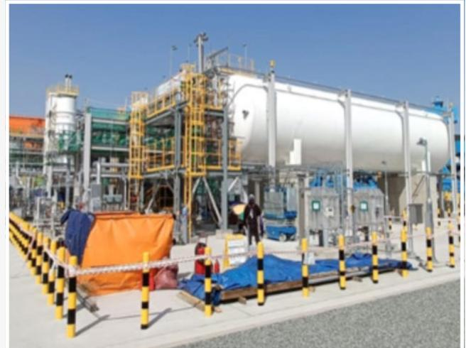
*Photos supplied by INOXCVA show four 311,000L liquid hydrogen tanks manufactured by INOXCVA in India for one of the largest prestigious projects for liquid hydrogen in South Korea. The liquid hydrogen is stored in vessels and is used for charging stations nationwide for buses, trucks and trams – with hydrogen as the ultimate clean fuel.*
